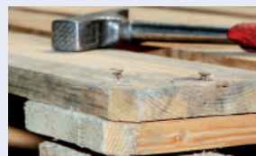
Hammering down projecting fastening elements
